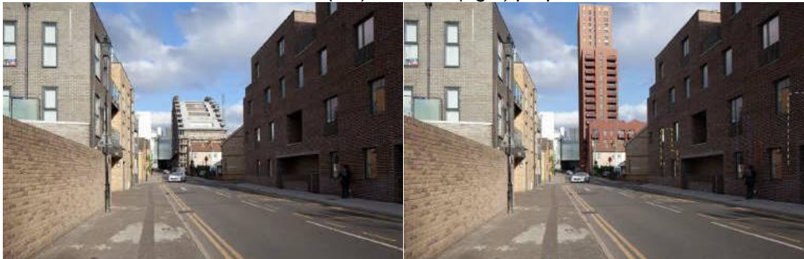
Figures 46 and 47: view from the north-western pavement of Drummond Road, opposite Maclean House towards the Site without (left) and with (right) proposal
