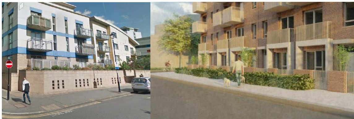
Figures 25 and 26: existing (left) and proposed view (right) of Frith Road elevation
